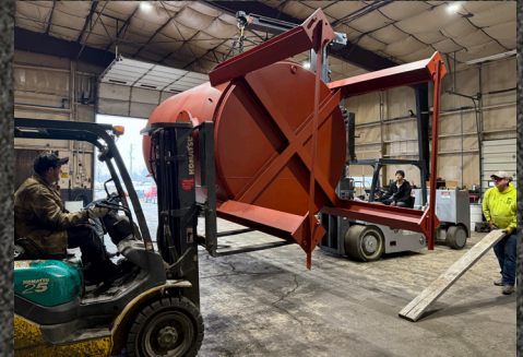
COOLING TANK INSTALLATION
